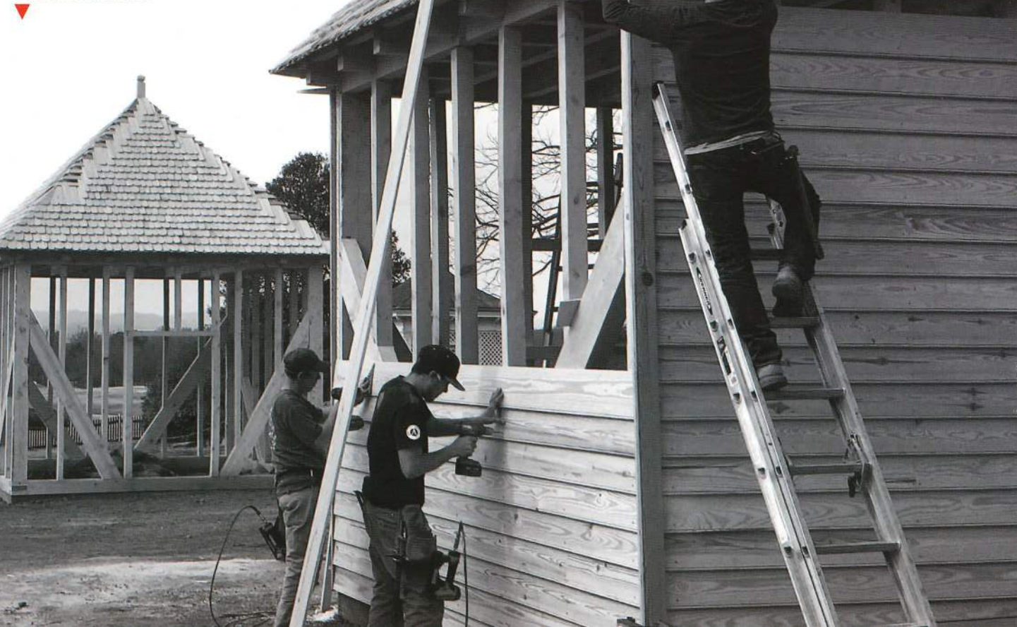
The team from Salvagewrights Ltd. reconstructing the South Yard smokehouses.
