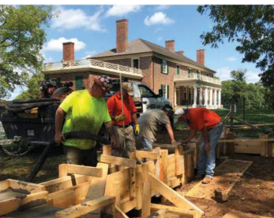
Laying the foundation for the Spinning House
